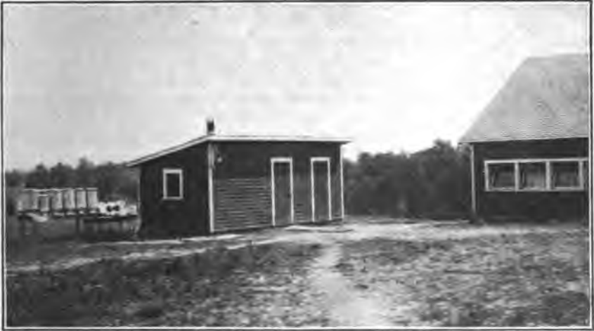
FIGURE 8.—A sanitary and convenient milk house, built according to plans recommended by the United States Department of Agriculture. This type of house is not expensive
